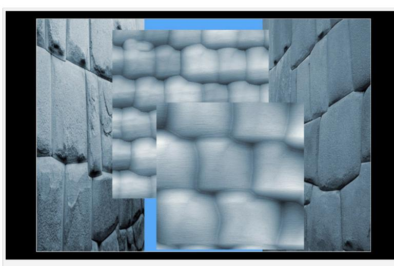
The survived wall fragments of splendid temples erected by the ancient Inca were built of large stone blocks with no mortars applied (shown in the image on the left and on the right). The stones are so precisely fitted that a knife blade can not be jammed between them. No one will ever confuse the stonework of the ancient Inca with any other.
